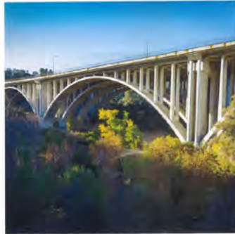
▲ A reinforced concrete bridge
